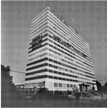
Figure 5: shows the image of a high building.
